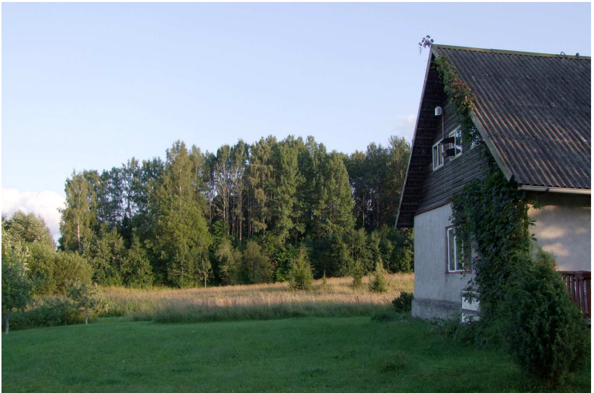
Figure A6.2. Cottage Tammemäe and the SIGMA air inlet in the center of the gable.
